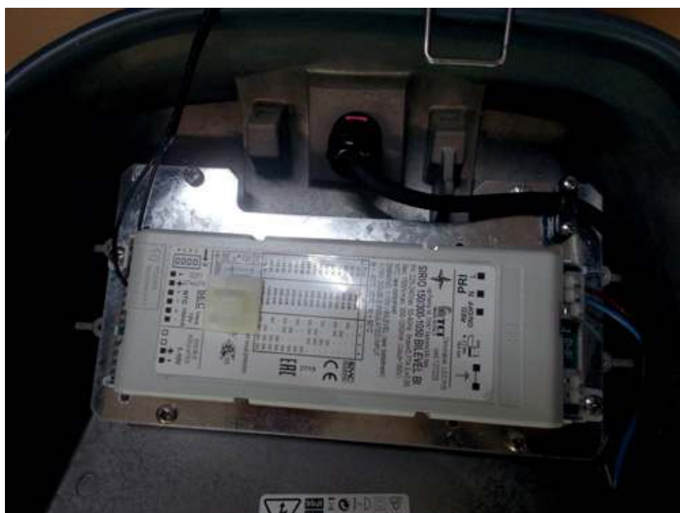
Pic.9: internal view
