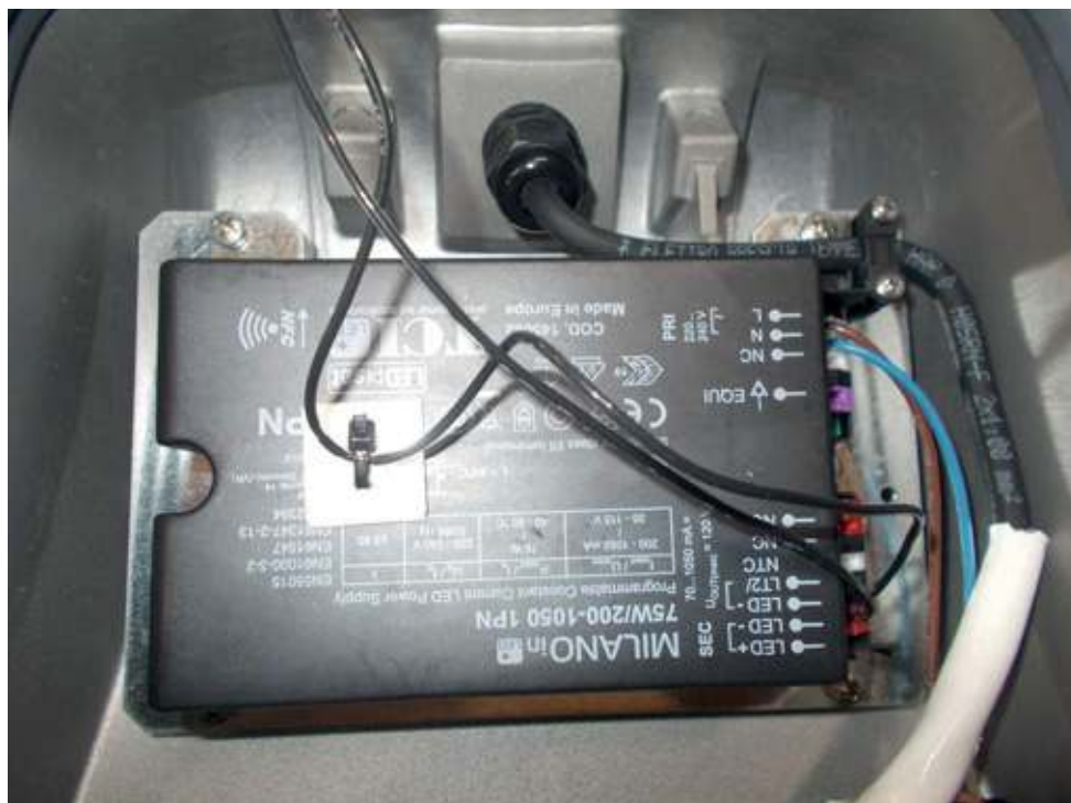
Pic.10: internal view
