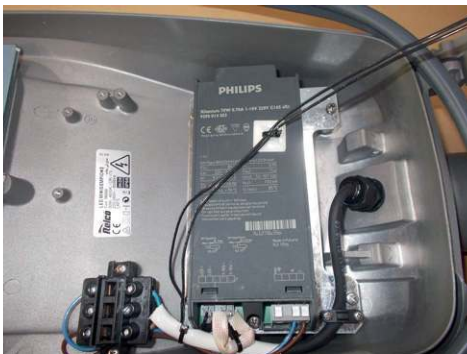
Pic.11: internal view
