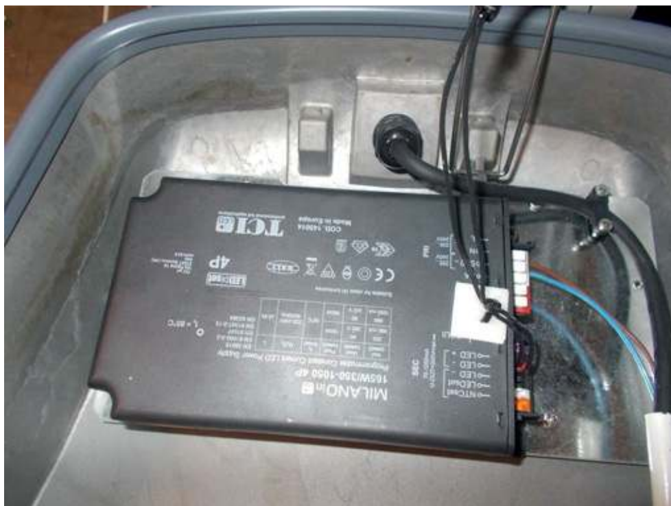
Pic.8: internal view
